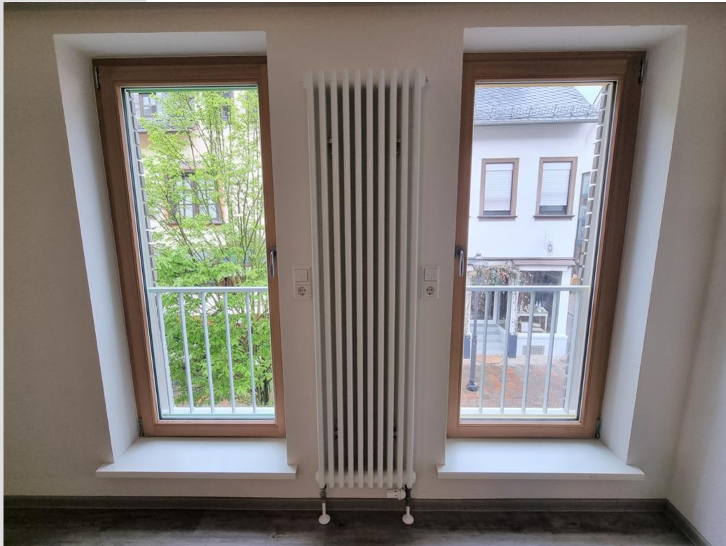
Detail Fenster (Personal)
